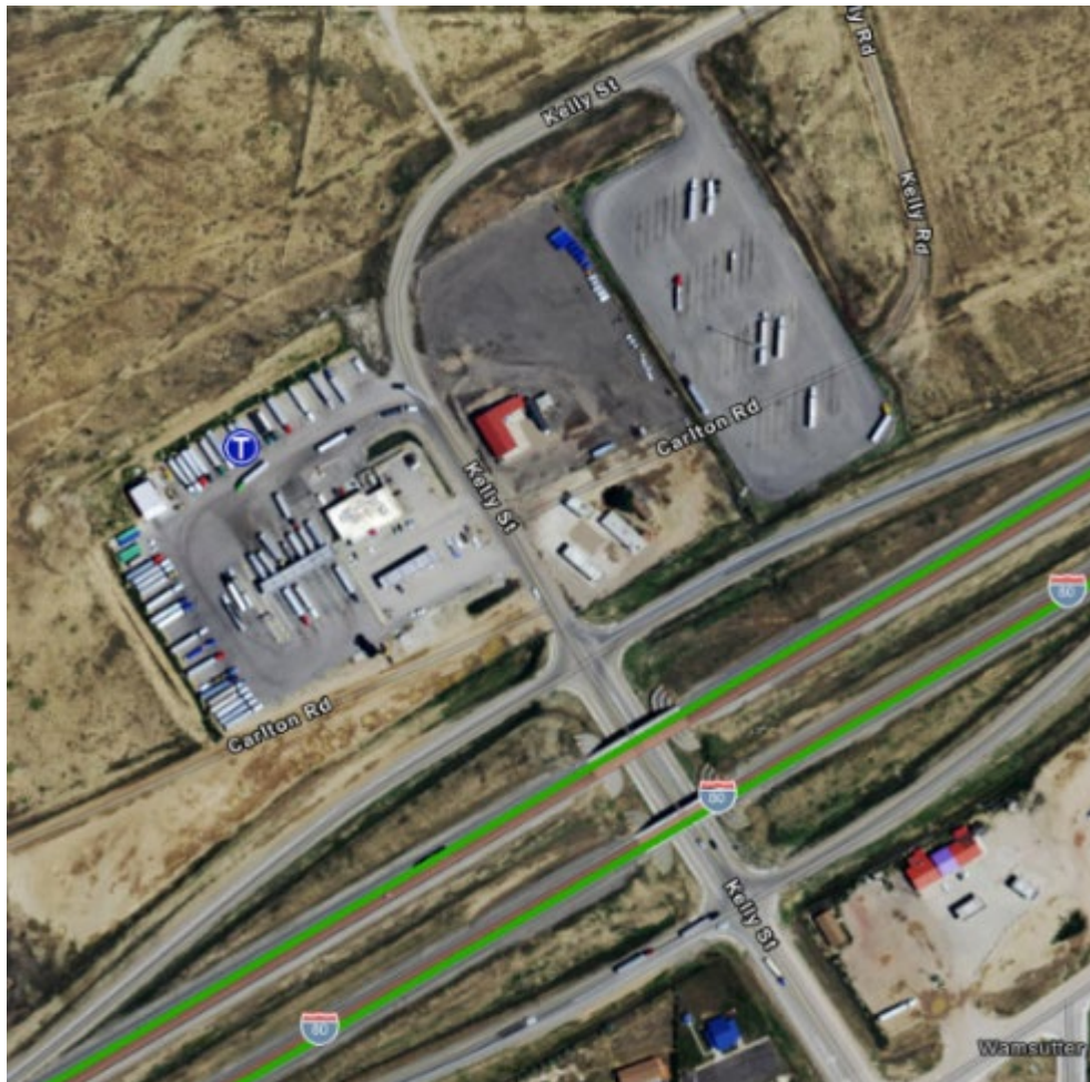
Figure 8: Aerial image of truck parking constructed by Wyoming DOT off of I-80. Wyoming DOT used a Truck Parking Facilities (TPF) Program grant to construct 43 truck parking spaces. Source: Google Earth.
