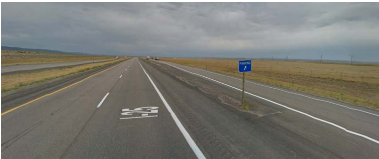
Figure 11: Street view of truck turnout area in Casper, Wyoming. Source: Map data ©2018 Google, DigitalGlobe.
