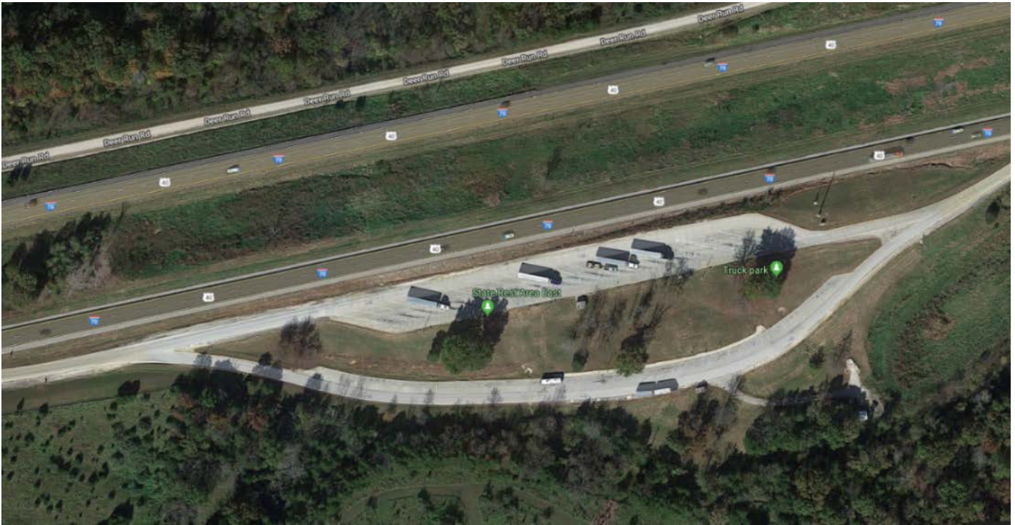
Figure 1: Aerial view of a Missouri rest area converted to provide truck parking. Source: Map data ©2018 Google, DigitalGlobe.
