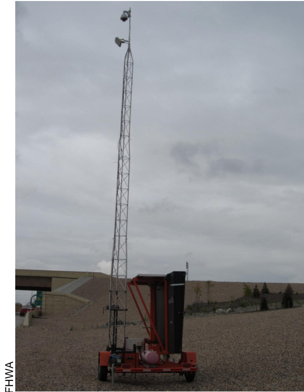
Figure 13. Photo. Temporary ITS Devices along I-15.
