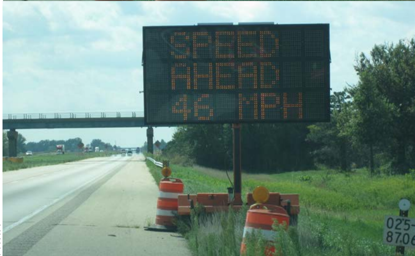
Figure 7. Photo. Messages Displayed on Portable CMS were Altered to be More Specific (Bottom) than what was Required in the Initial Special Provision (Top).
