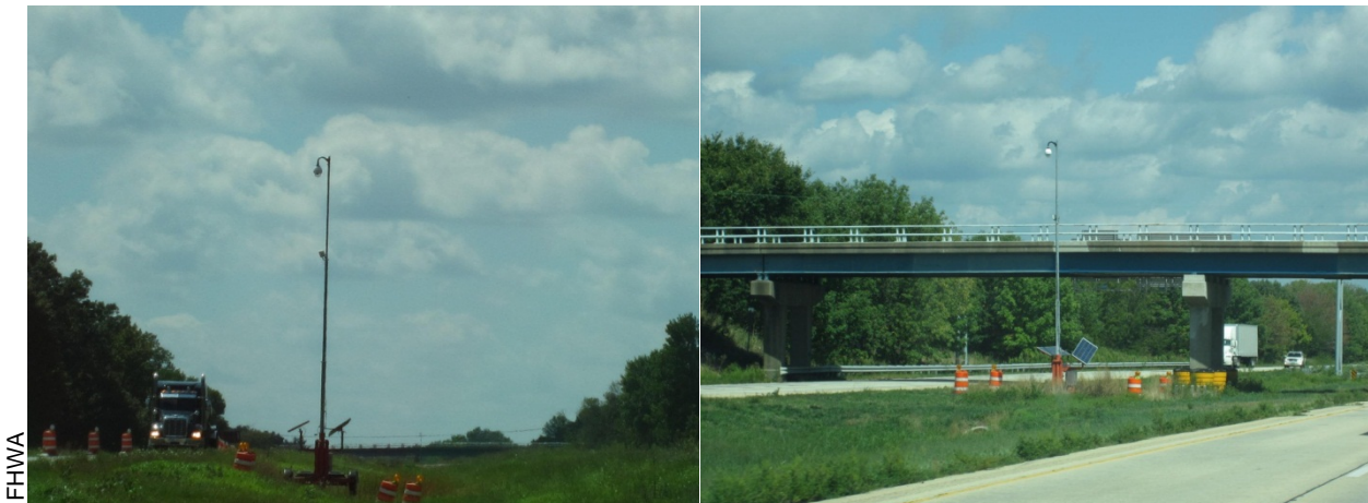
Figure 4. Photo. Temporary, Solar-Powered Traffic Detection and Camera Systems.
