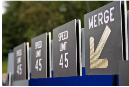
Figure 3. Photo. Example of overhead dynamic speed limit signs.
