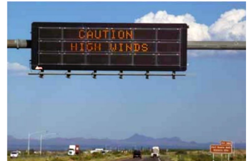
Figure 2. Dynamic message sign with warning message. (Source: Arizona Department of Transportation)
