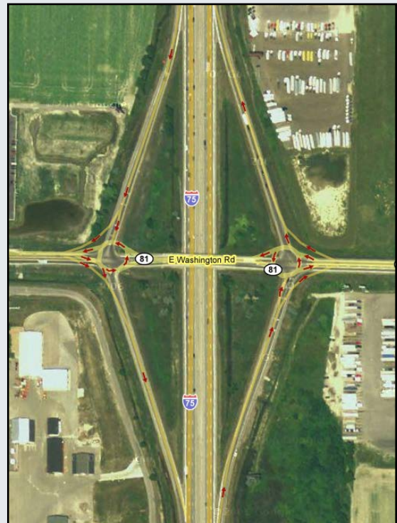
Roundabout Solution at I-75/M-81
