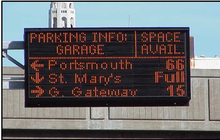
Figure 2-3. Dynamic Message Signs Will Guide Drivers to Available Parking in San Francisco
