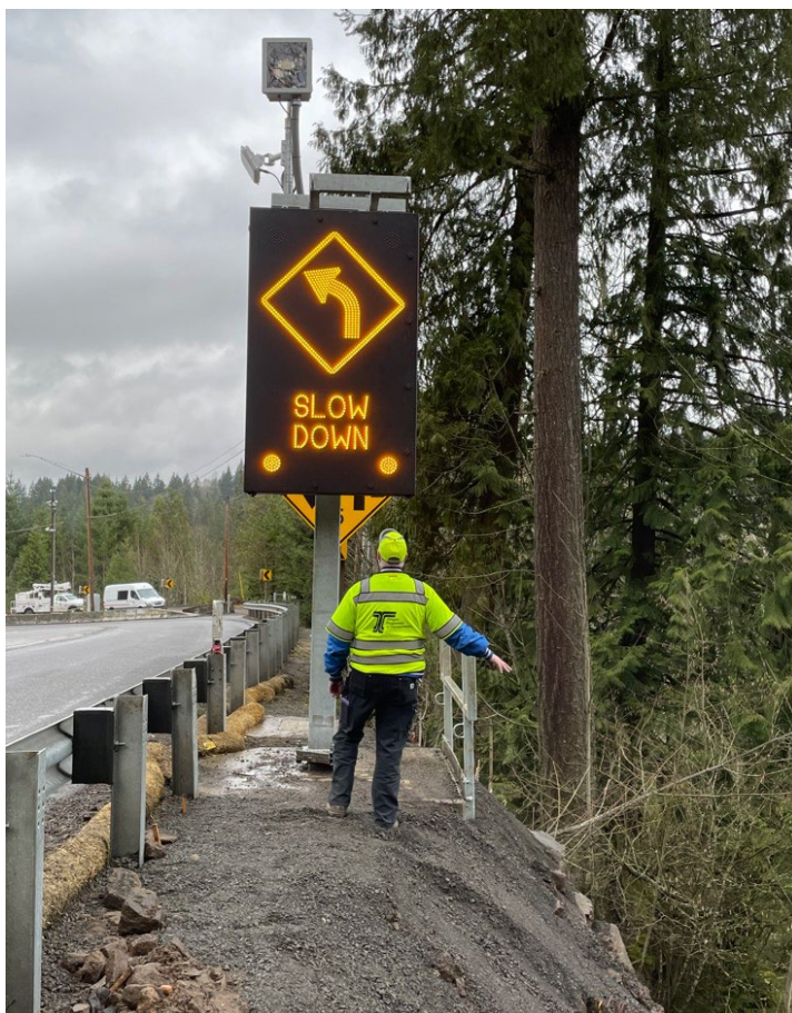
CURVE WARNING SIGN INSTALLATION
