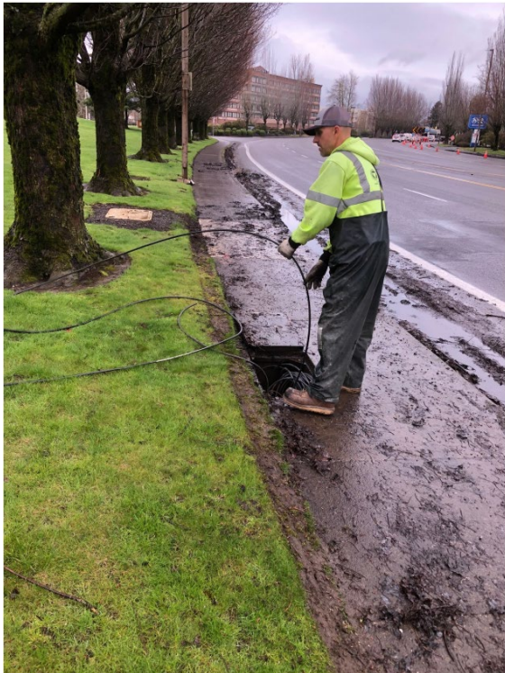
FIBER OPTIC INSTALLATION
