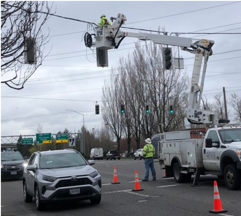
LEFT: INSTALLATION OF FIBER OPTIC CABLE; RIGHT: TRAFFIC SIGNAL CONTROLLER UPGRADES
