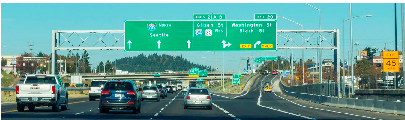
I-205 NB AUXILIARY LANE
