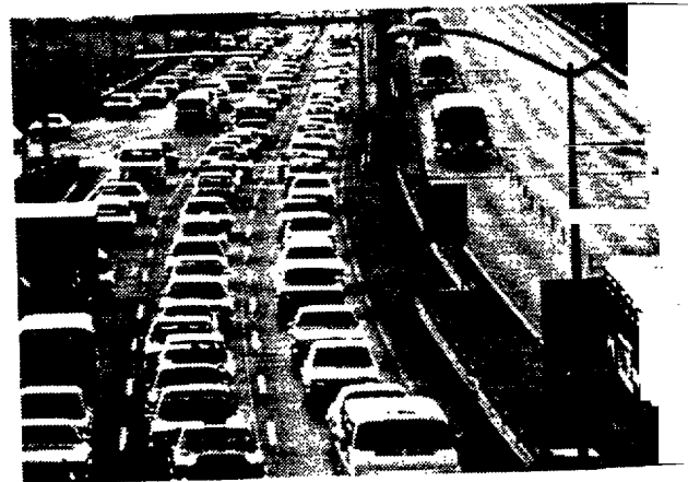
Contraflow Lane, Gowanus Expressway, New York City
