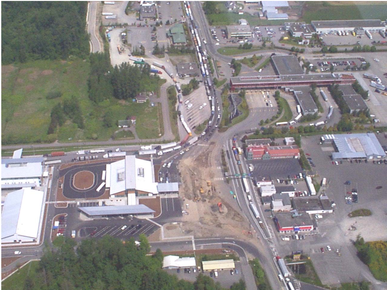
Figure 2. Blaine Border Crossing (looking North)
