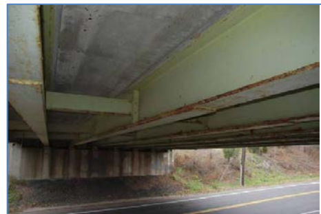
Source: Connecticut DOT/USDOT FHWA
