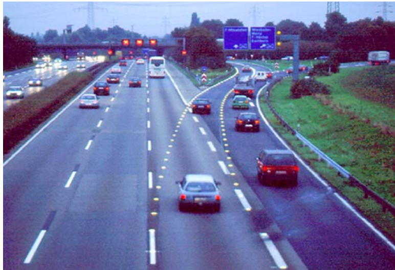
Figure 7. Junction Control at an Exit with Hard Shoulder Running
