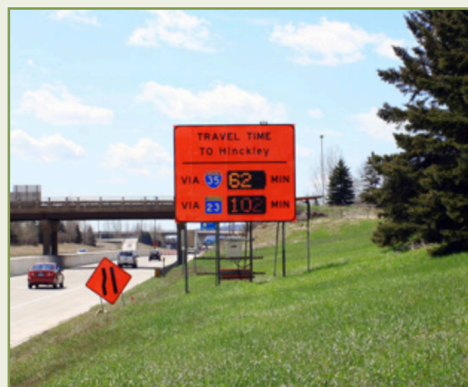
Travel Time Sign Located Near 40th Avenue on I-35 in Duluth
