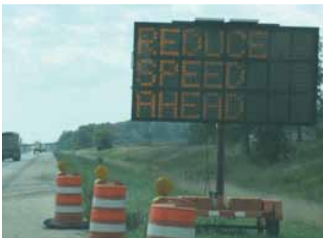
Figure 22. PCMS messages were modified from a generic message (left) as stated in the contract to a more specific message (right).
