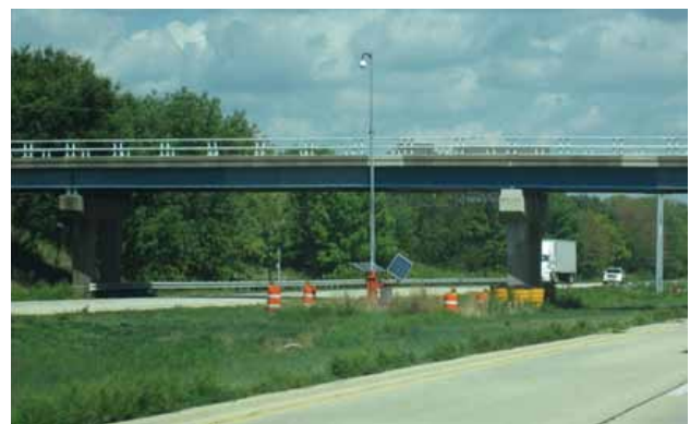
Figure 2. Temporary, solar-powered vehicle detection and camera systems.
