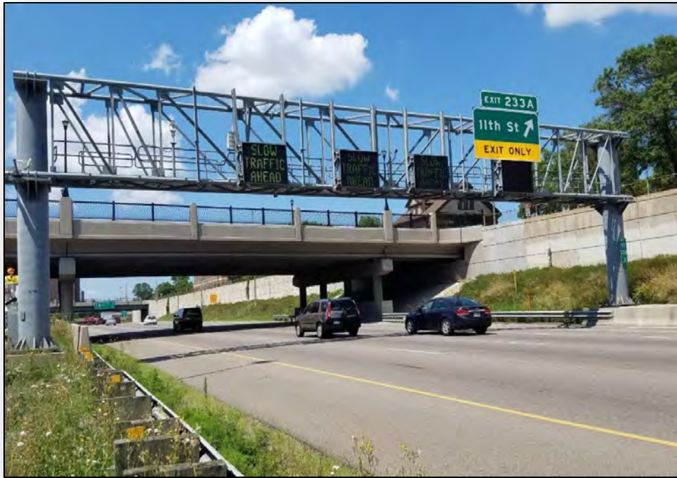
Figure 13. Photo. Queue warning message boards on I-94, Minneapolis, Minnesota (Source, MnDOT).
