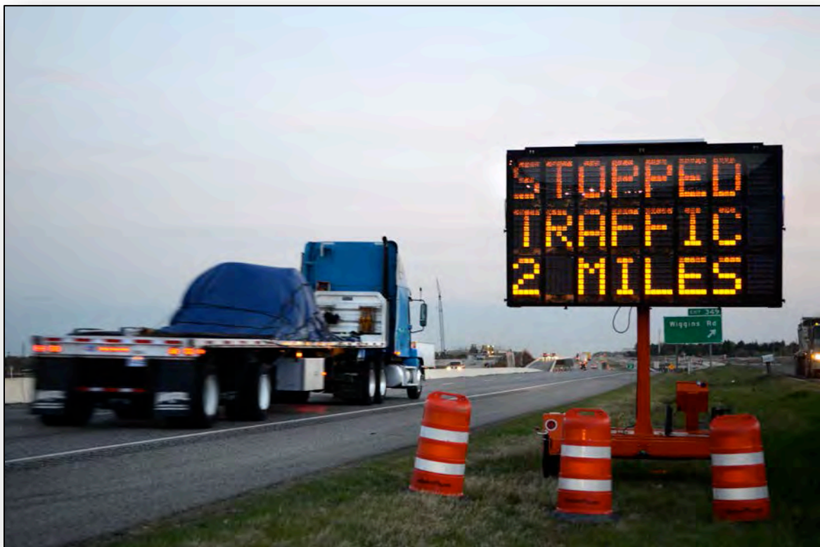
Figure 12. Photo. Queue warning work zone application on I-35, Waco, Texas (Source: TTI).
