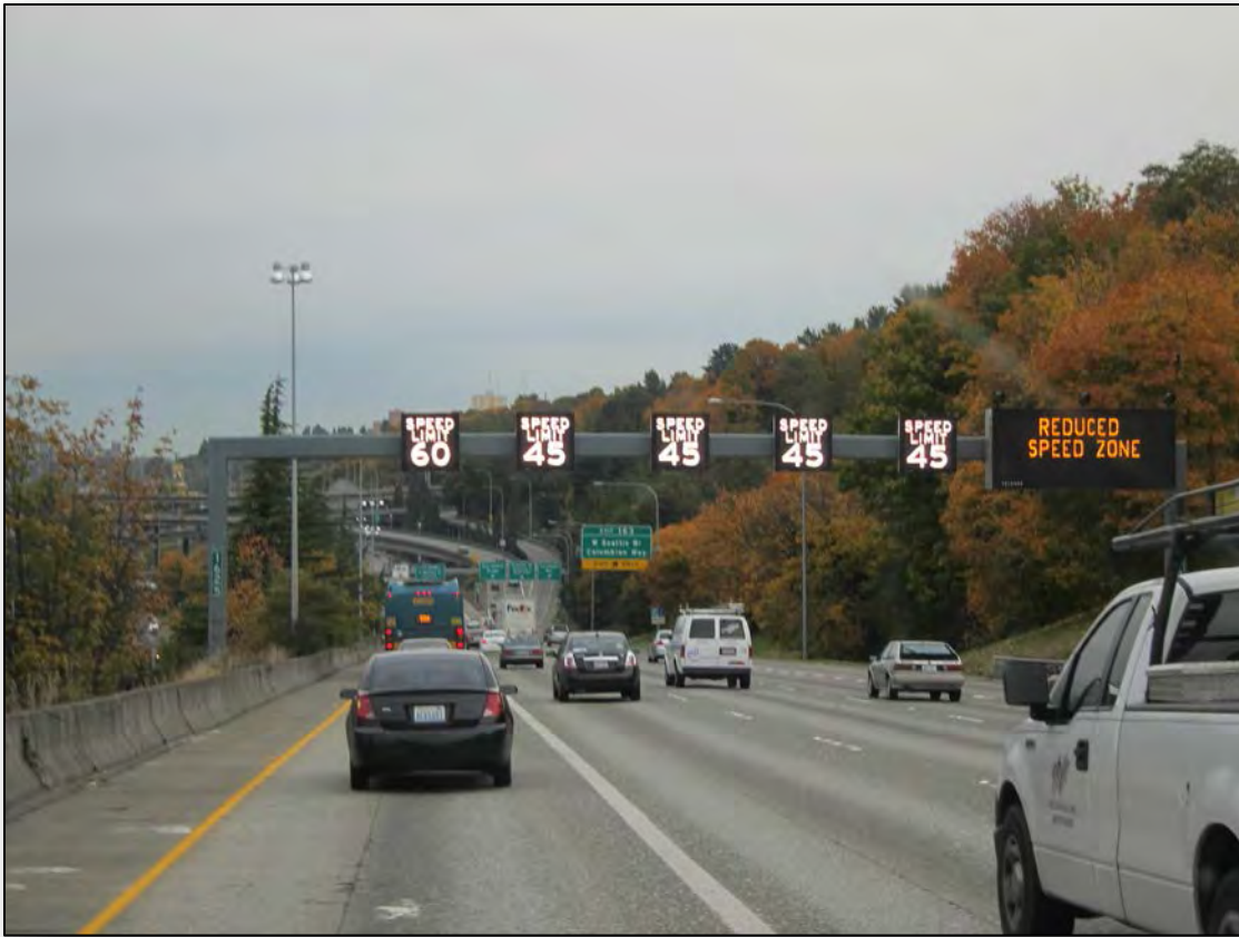
Figure 1. Photo. ATM installation on I-5, Seattle, Washington (Source: Texas A&M Transportation Institute [TTI]).
