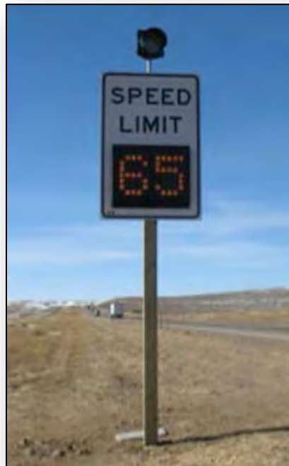
Figure 3. Photo. VSL sign in Wyoming (Source: WYDOT).
