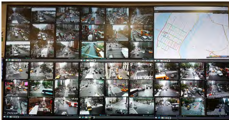
Figure 7. Photo. ATSC camera images in New York City (Source: New York City Department of Transportation).
