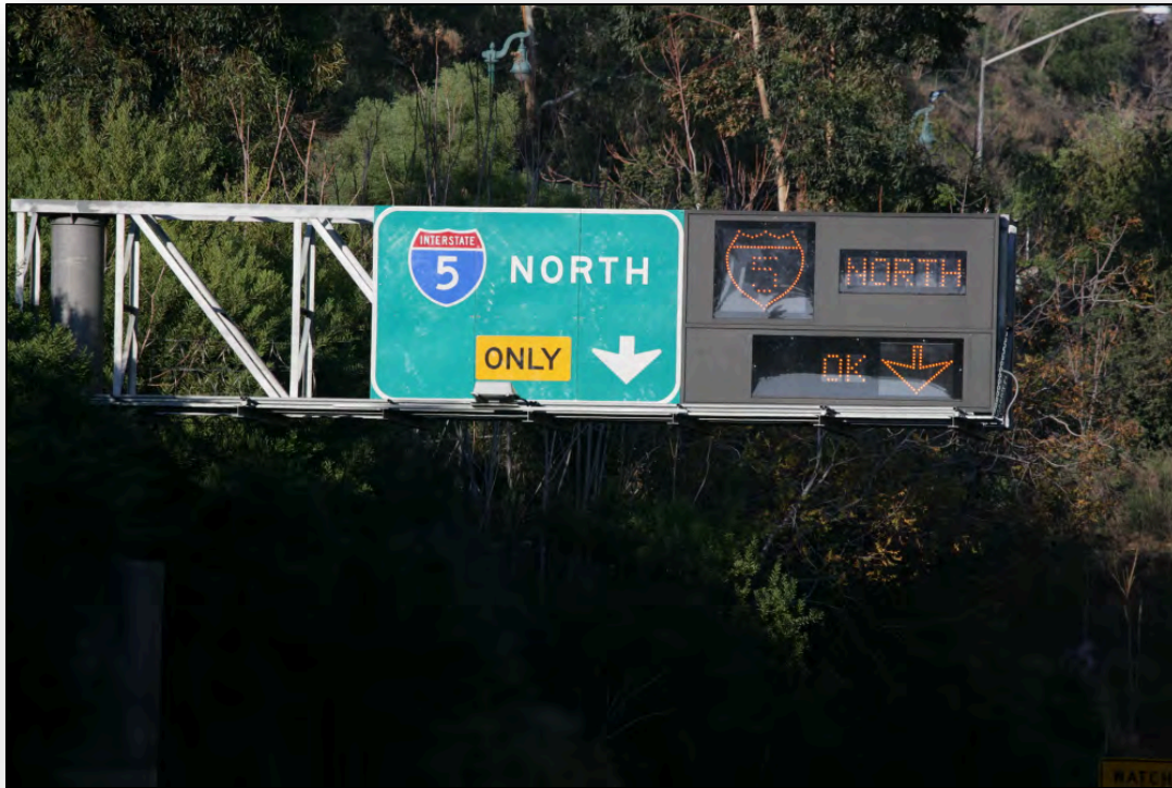
Figure 8. Photo. Dynamic junction control signing on SR 110 (Pasadena Freeway), Los Angeles, California (Source: Caltrans).
