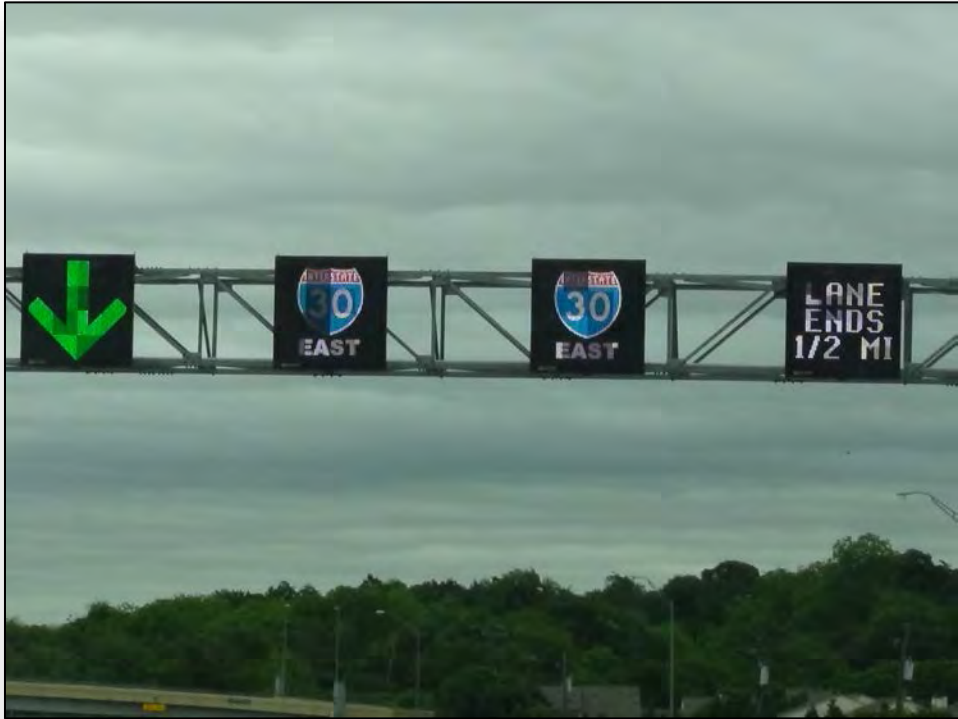
Figure 10. Photo. DLUC application on I-30 in Texas (Source: TTI).
