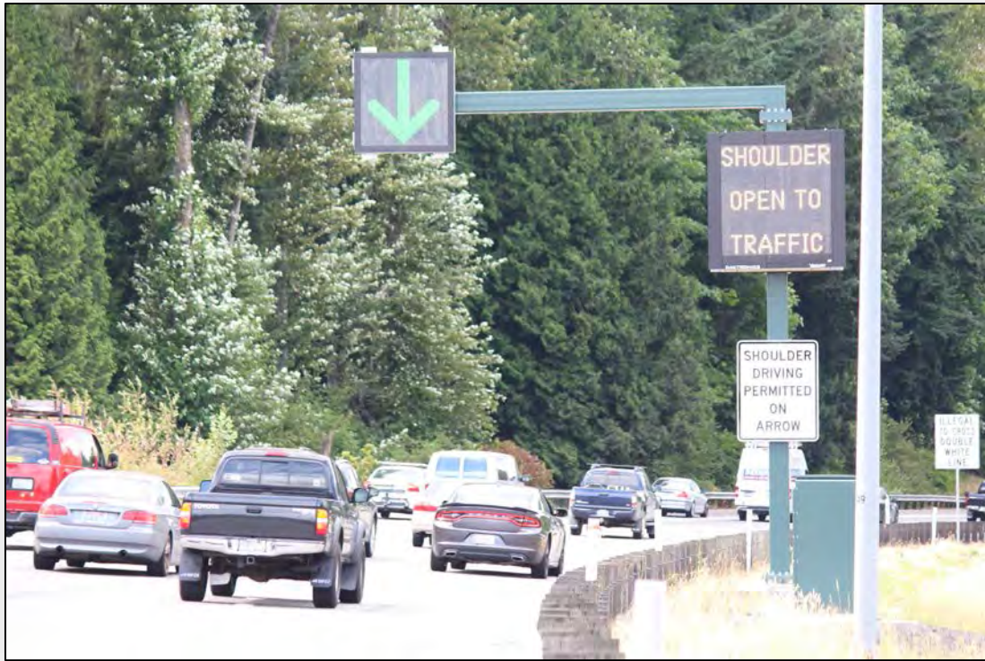
Figure 11. Photo. DShL application in Seattle, Washington (Source: WSDOT).
