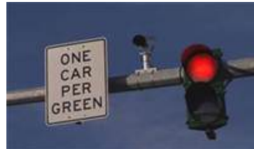
Figure 22. A ramp meter. (Source: Federal Highway Administration.)
