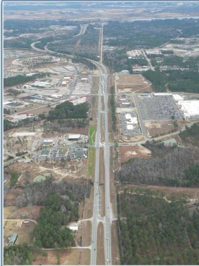
Figure 17. Photo. U.S. Route 17 restricted crossing U-turn intersection corridor in Leland, North Carolina. (Source: Federal Highway Administration, Restricted Crossing U-turn Informational Guide.)
