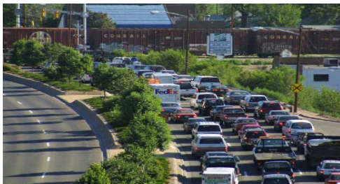
Figure 20. Traffic backed up on northbound Wadsworth prior to the project. Restaurant (blue roof) had to be relocated.
