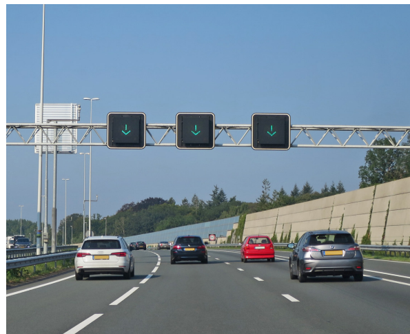
Figure 51. Photo. Dynamic shoulder lane open on the left.
