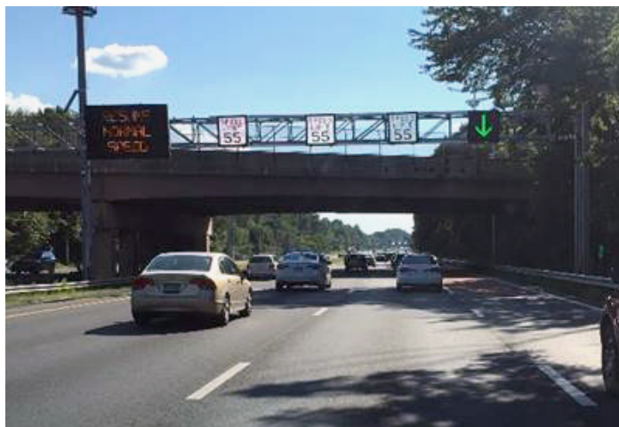
Figure 3. Photo. A lane-use control sign (on the far right side) indicates whether the shoulder is open or closed to traffic.
