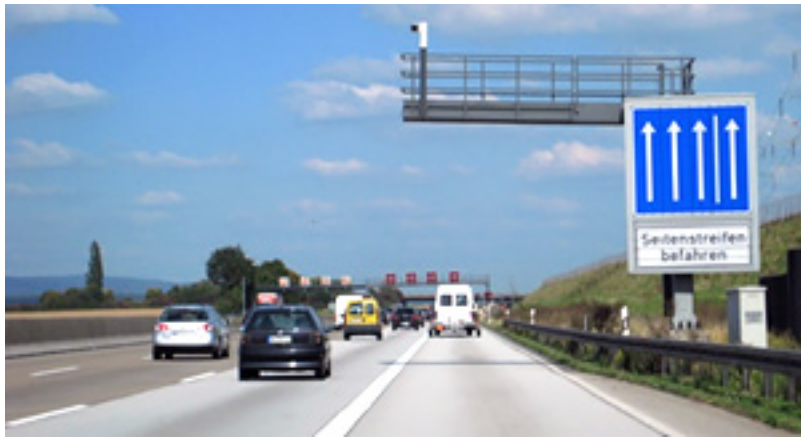
Figure 49. Photo. Dynamic shoulder lane open.
