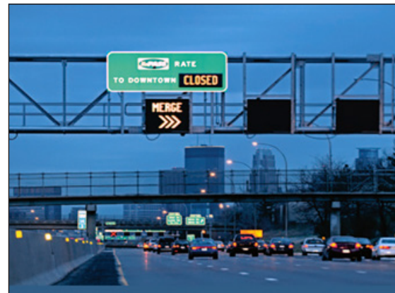
Figure 42. Photo. Dynamic shoulder lane closed.
