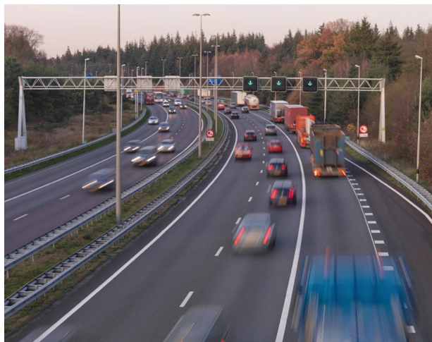
Figure 50. Photo. Dynamic shoulder lane open on the right.
