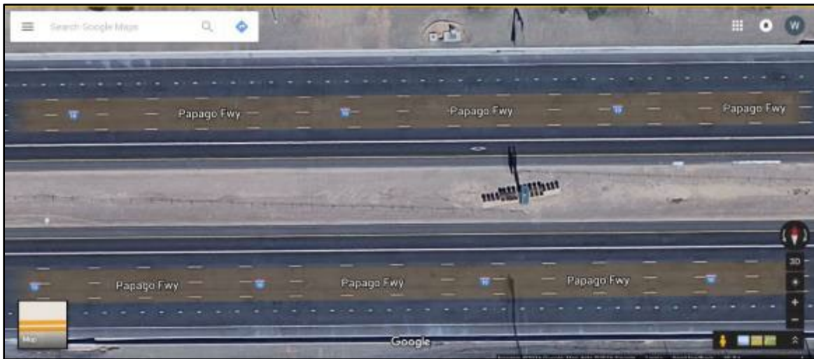
Figure 32. Photo. Aerial view of Corridor 3.
