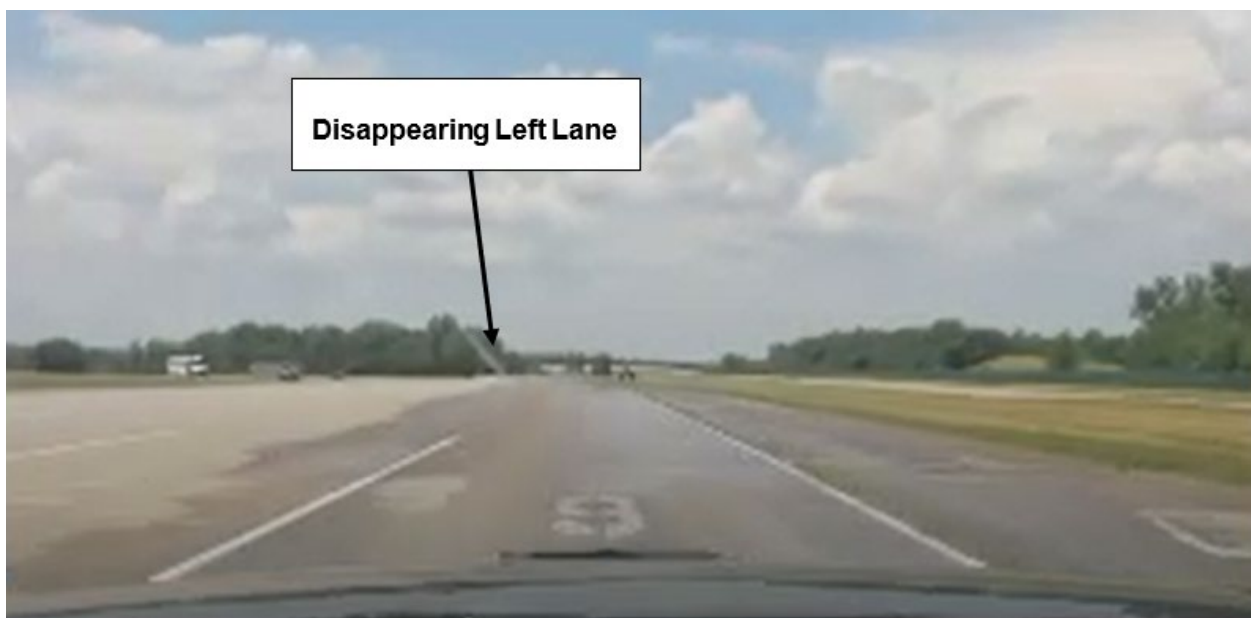
Figure 18. Photo. Test vehicle point of view depicting disappearing left lane line on lane 6.
