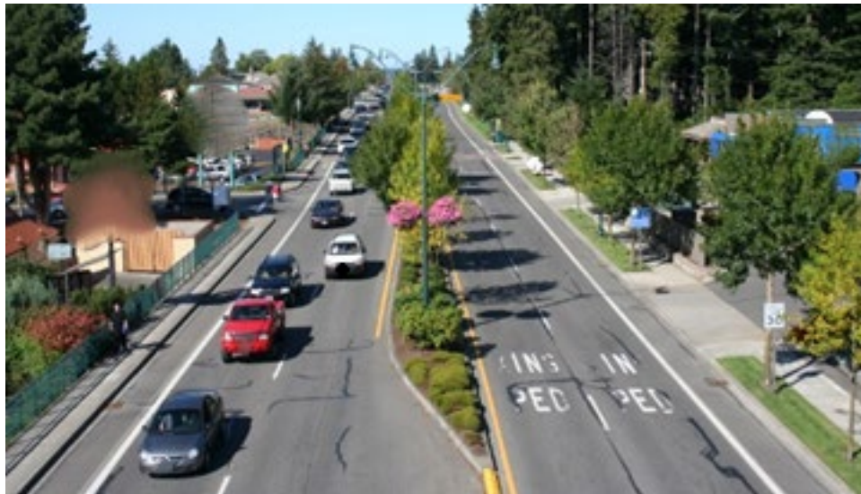
Figure 5. Photo. Bridgeport Way after access management project. Source: National Academies of Sciences, Engineering and Medicine. 4
