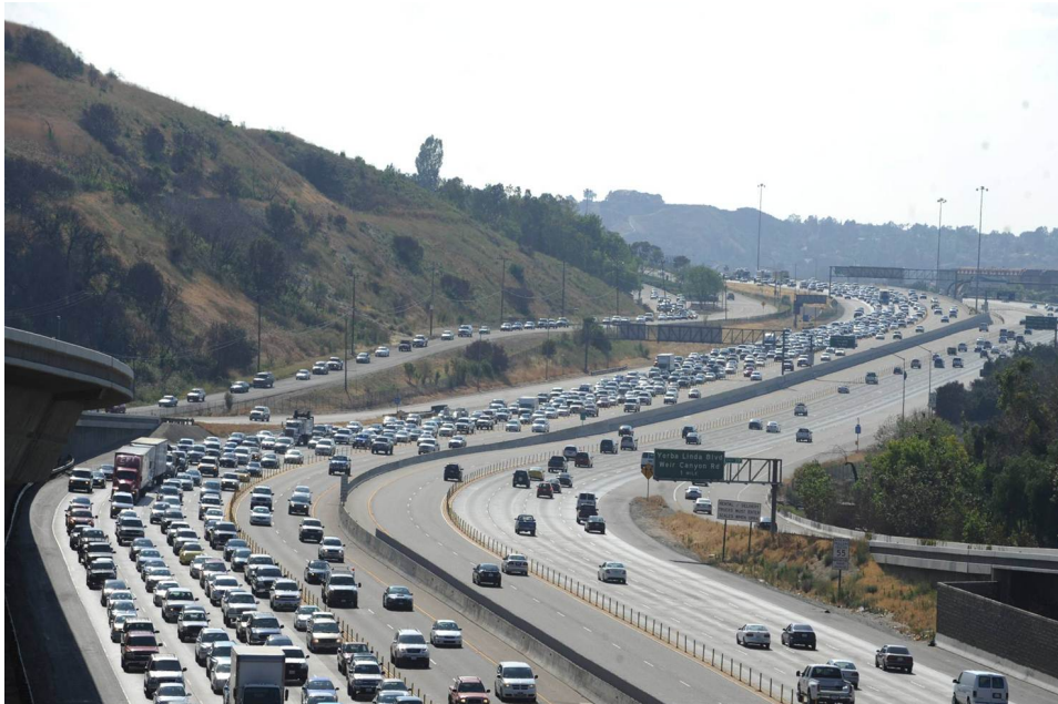
Source: Orange County Transportation Authority Figure 4. Photo. Buffer-Separated Express and General-Purpose Lanes in Orange County, CA.
