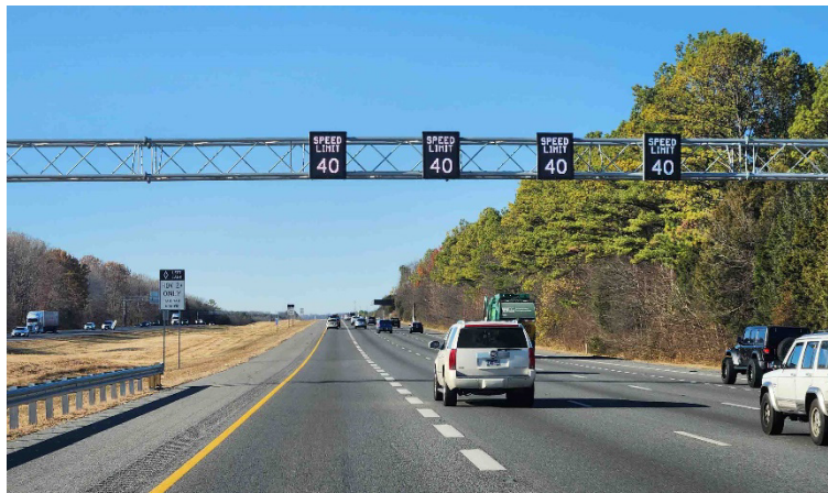
Figure 4. Variable speed limits above Tennessee I-24.
