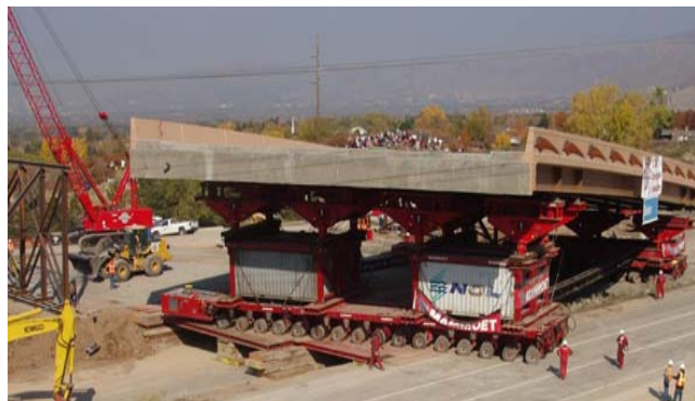
Bridge Move with SPMT (Source: FHWA Highways for Life)
