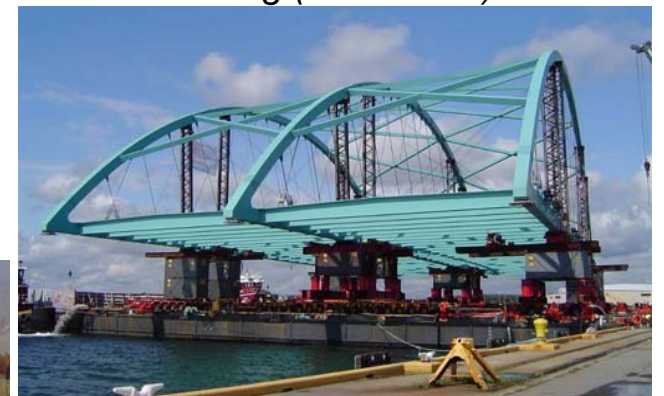
Bridge Move with SPMT (Mammoet)
