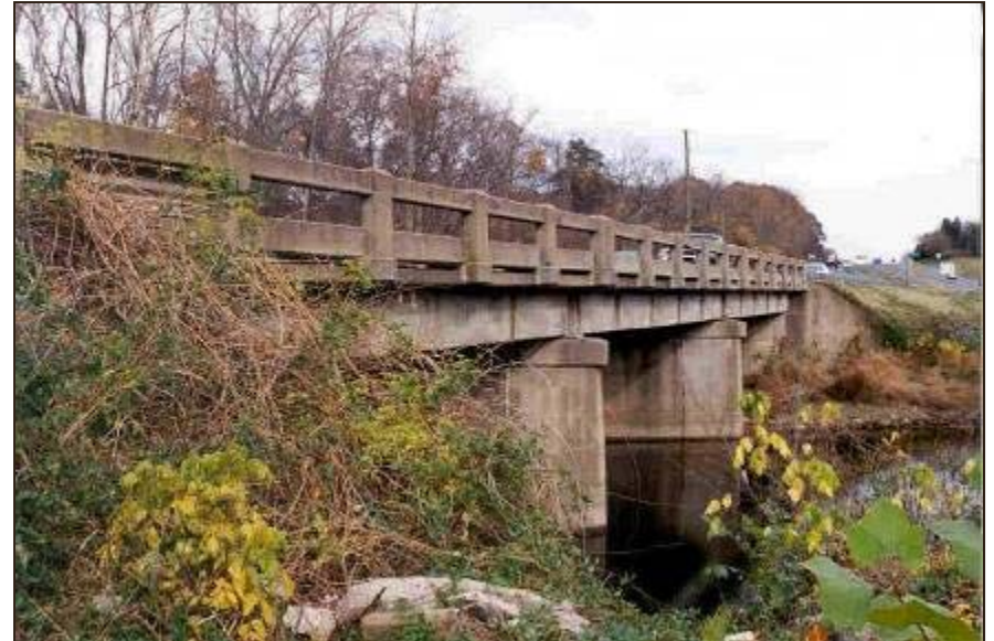
East side view of SBL bridge prior to construction
