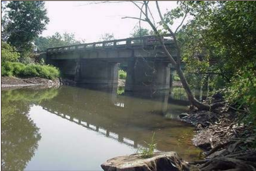
West side view of SBL bridge prior to construction
